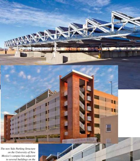
on the University of New Mexico's campus lies adjacent to several buildings on the National Register of Historic Places, requiring the parking facility pay homage to that aesthetic while providing desperately needed parking space. A total precast concrete structural system helped it meet all of its aesthetic, functional, construction, and budget goals.
