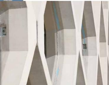
The new Nanotechnology Research & Application Center at Sabanc University in Turkey features an innovative use of precast concrete as a structural lattice that symbolizes the work accomplished at the facility. The precast concrete lattice consists of 53 modules, each 24 feet high and 20 inches thick, with a layer of insulation sandwiched between two layers of concrete.
